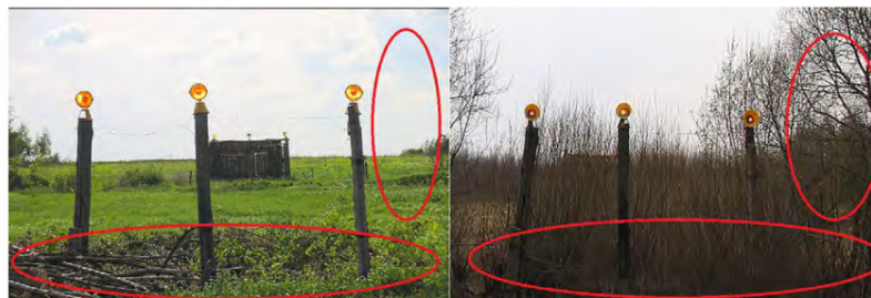
Fig. 21. SMOLEŃSK NORTH – difference in tree stands in „A” area – approach path lamps, about 600 m from RWY THR 26
