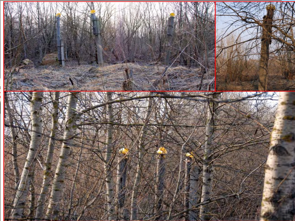
Photo 20. Navigation lamps obscured by trees and shrubs
